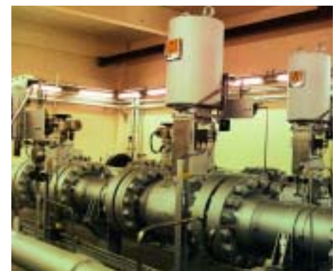
HIPPS valve 16" ANSI 1500 lbs in German compressor station
