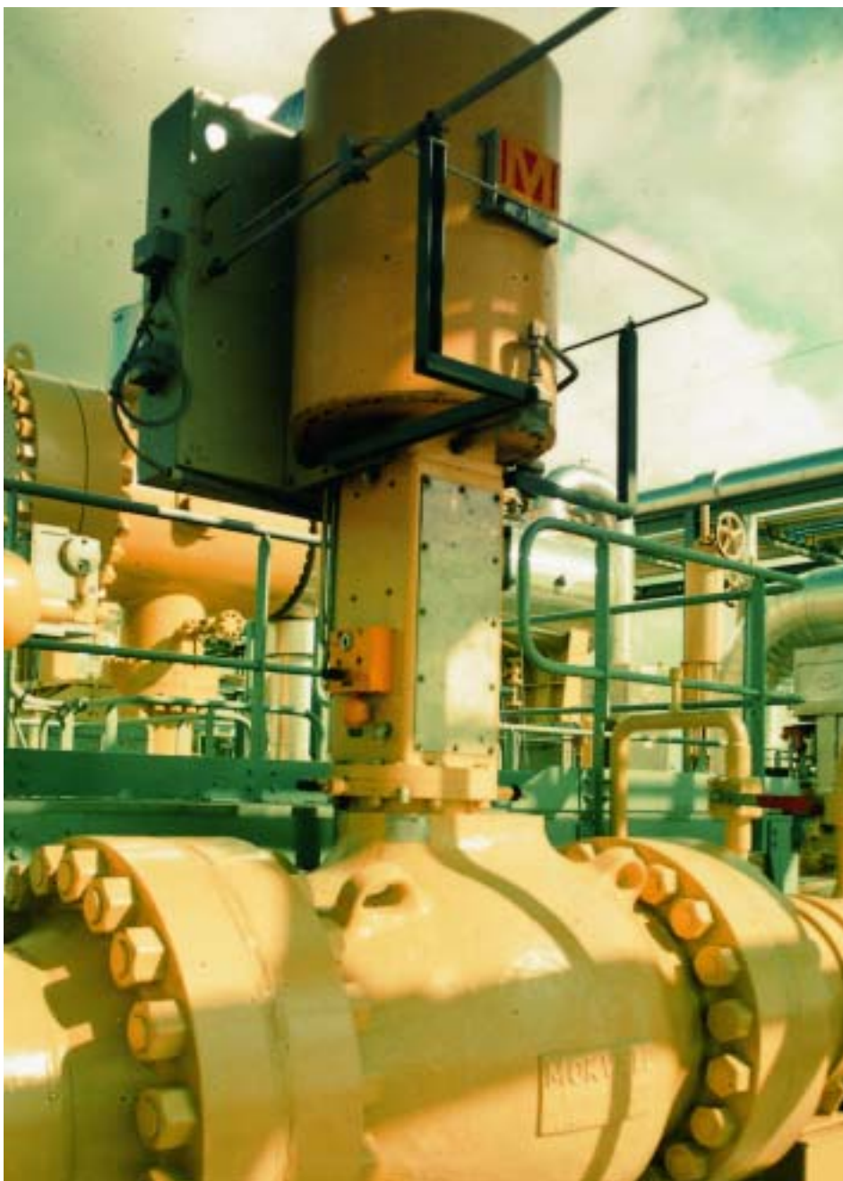
HIPPS valve 16" ANSI 1500 lbs in German compressor station
