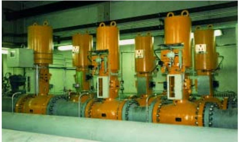
*pressure control valves 20" ANSI 600 lbs and safety slam shut valves
