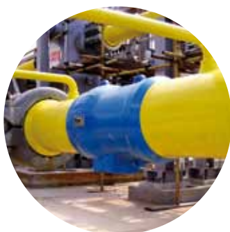
20" / ASME 2500 Axial Check Valve
