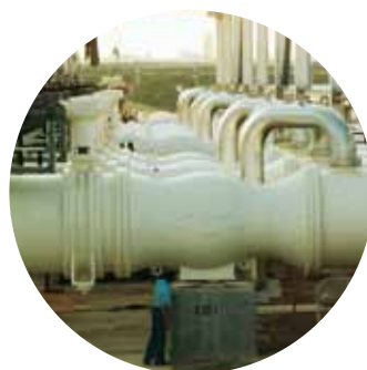
72" / ASME 175 Axial Check Valve
